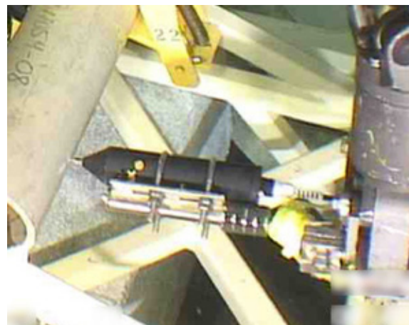
CATHODIC PROTECTION SURVEY
