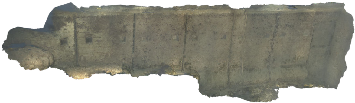
3D model - Quay wall inspected with Hydro 100
